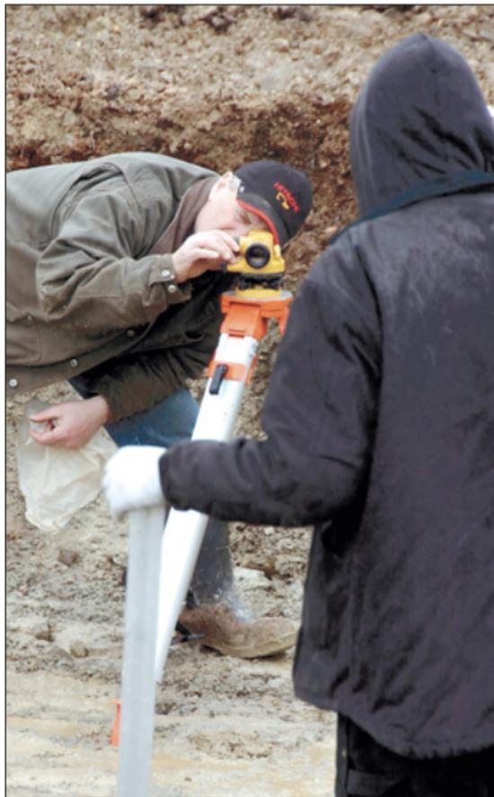
**Bruce Guest (left) takes measurements to check if the ground is level in a hole for a new house foundation on New Pennywell Road. At right is co-worker Craig Duke. Both are employees of Miller Equipment.** — Photo by Keith Gosse/The Telegram
